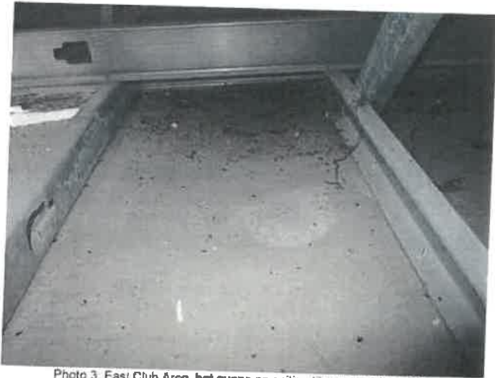
Photo 3: East Club Area, bat guano on ceiling tiles near column G7.
