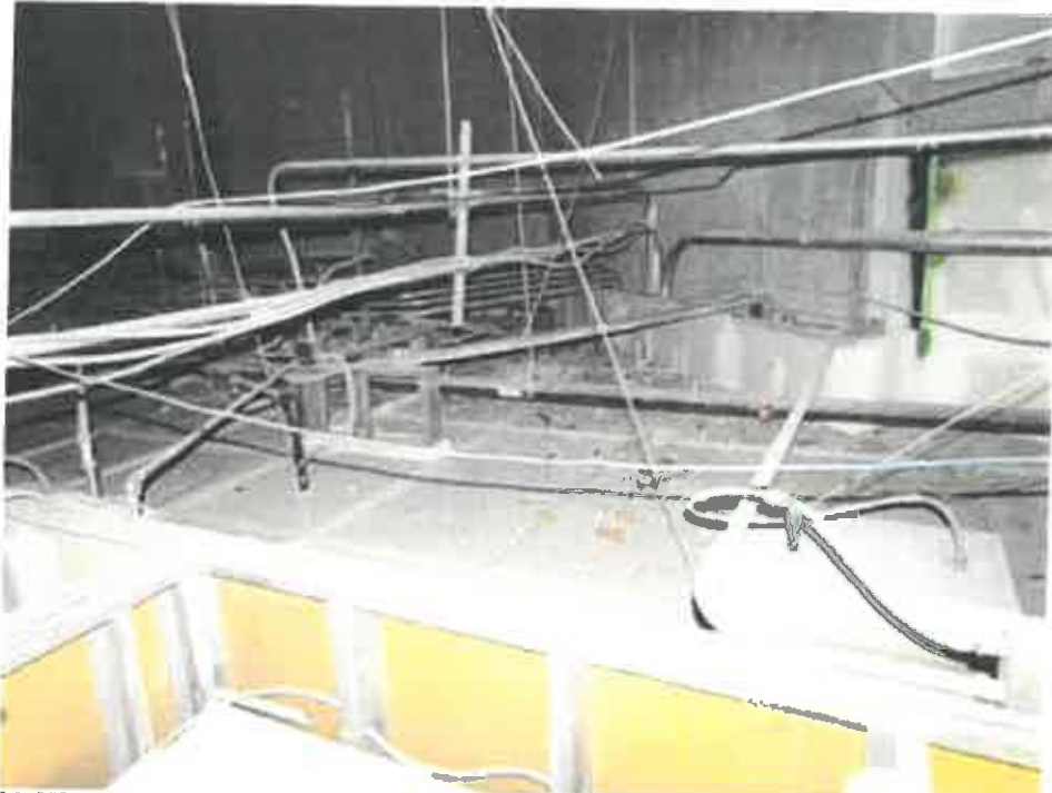
Photo 11: West Club Area, debris mixed with bat guano on ceiling tiles above concession stand near column lines G & H 37.4
